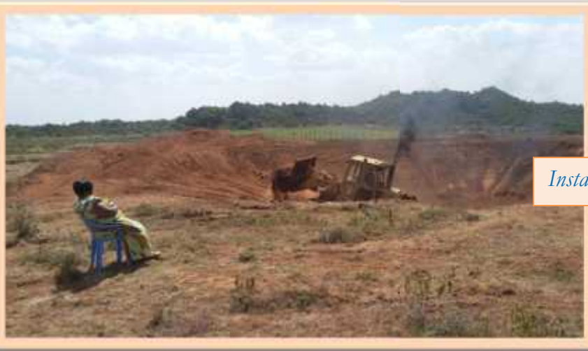
The project supervisor herself positioned to get the job done
